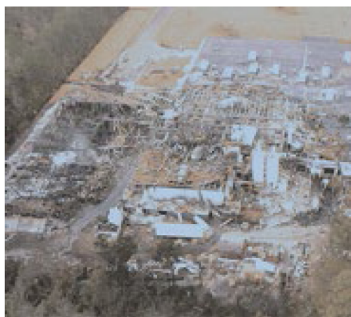
A pharmaceutical plant after a dust explosion.
